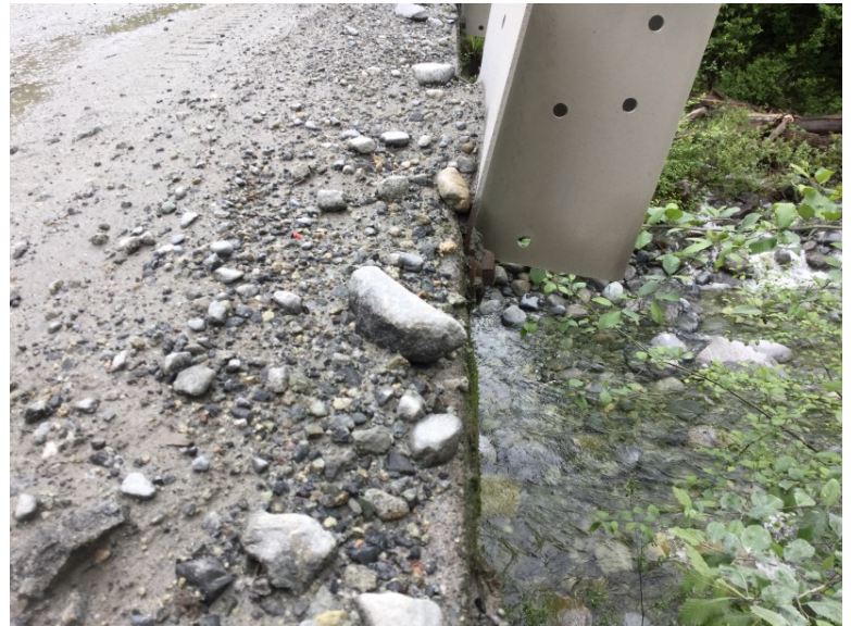
Guard Rail at downstream right bank
