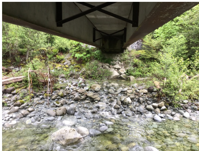
Left Bank Abutment when facing downstream
