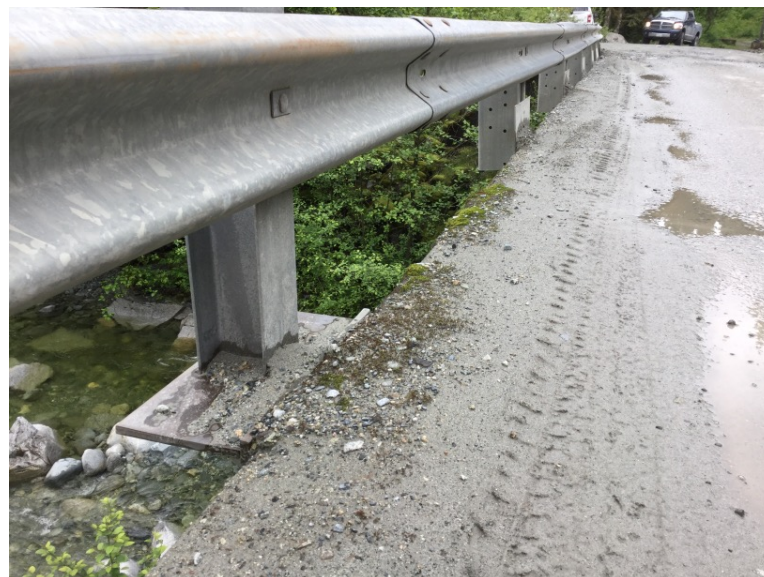
Downstream risers are different at downstream end
