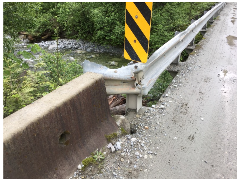
Guardrail condition at downstream left bank
