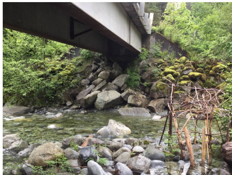
Right Bank Abutment when facing downstream
